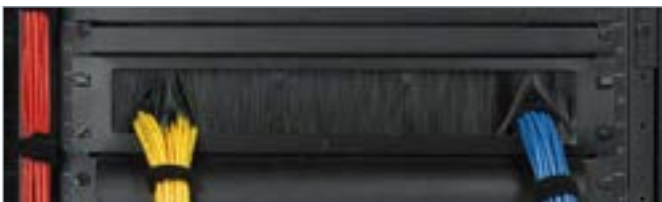
Brush strips allow routing of cables through the panel (Model: ETN-CMBPBRSH1U).
