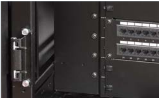
Vertical blanking panels seal open spaces and prevent bypass airflow in areas that are traditionally difficult to seal. They can also be adapted for cable management.
